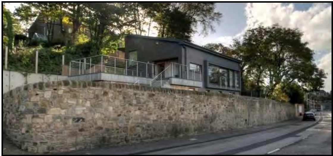
Figure 17c: Contemporary dwellinghouse at 84 Lower Granton Road
